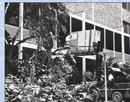
The delivery of the Scientific Data Systems (SDS) Sigma 7 computer to Boelter Hall at UCLA in 1967. SDS machines were early adopters of integrated circuits and silicon transistors; yet, despite this, their machines still contained considerable heft. To deliver this unit, a hole was cut into the outside wall of the building, where a forklift elevated the machine to its destination. (Courtesy of the UCLA Samueli School of Engineering)
